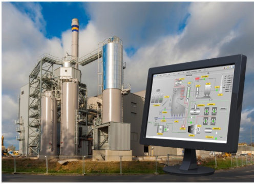
Picture 3: The combined heat and power station is monitored via the PMSXpro process control system from ME-Automation Projects.
